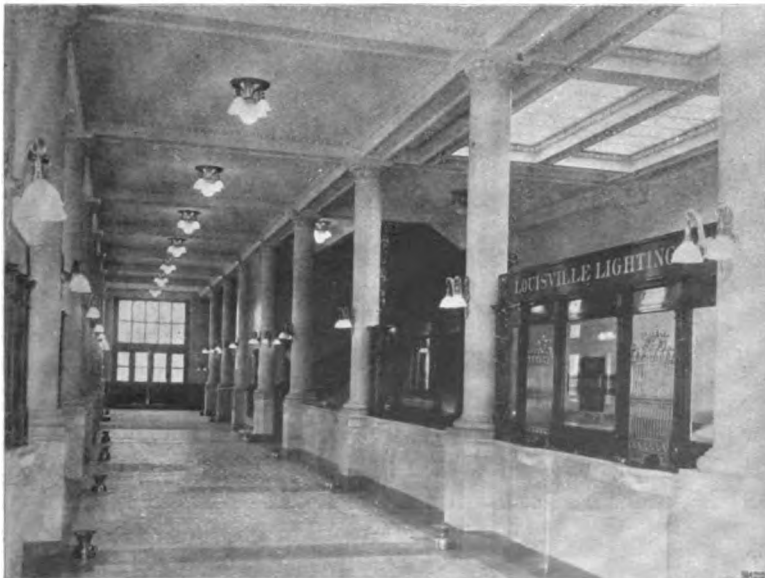
Offices of Louisville, (Ky.) Lighting Company.—An Attractively Lighted Corridor. Showing Combination of Globes and Bell-Shaped Reflectors.
